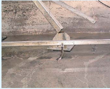
AVMS-Vibrations- schaden
